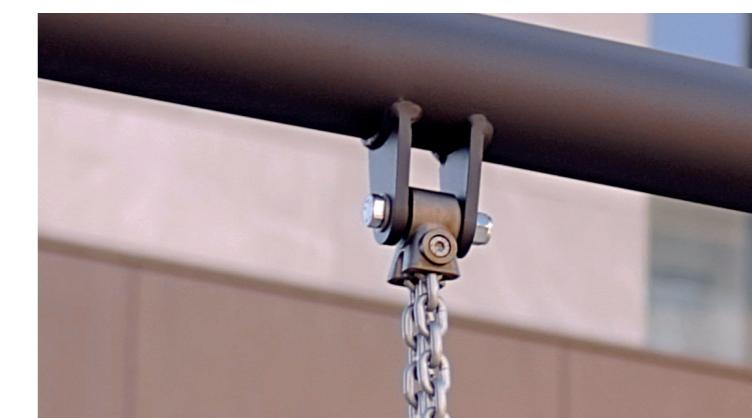
**Robot joint is a custom-designed high durability swing joint that also eliminates any figder entrapment issue. The swing upper joint mechanism was produced with the precision casting technique Between the two ears welded on the swing carrier pipe, rigid bedding to be fixed with M12x80 bolts and a Teflon bearing should be used to prevent abrasions.**
