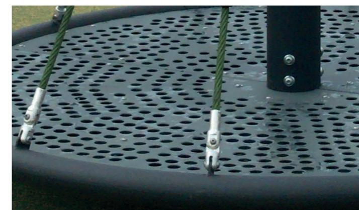
**Platforms are made of plastic-coated steel sheets which are decorated with drainage and holes. Plastic coating provides further protection against falls and weather conditions.**
